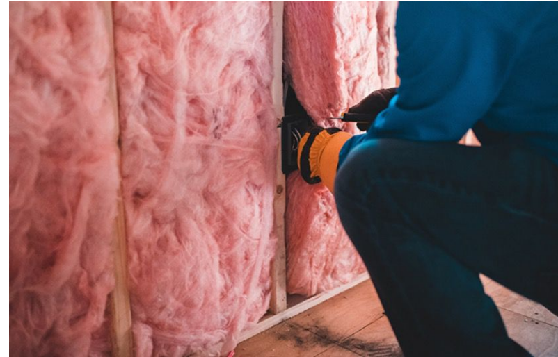
Adding insulation into a house. Source: RIBA
